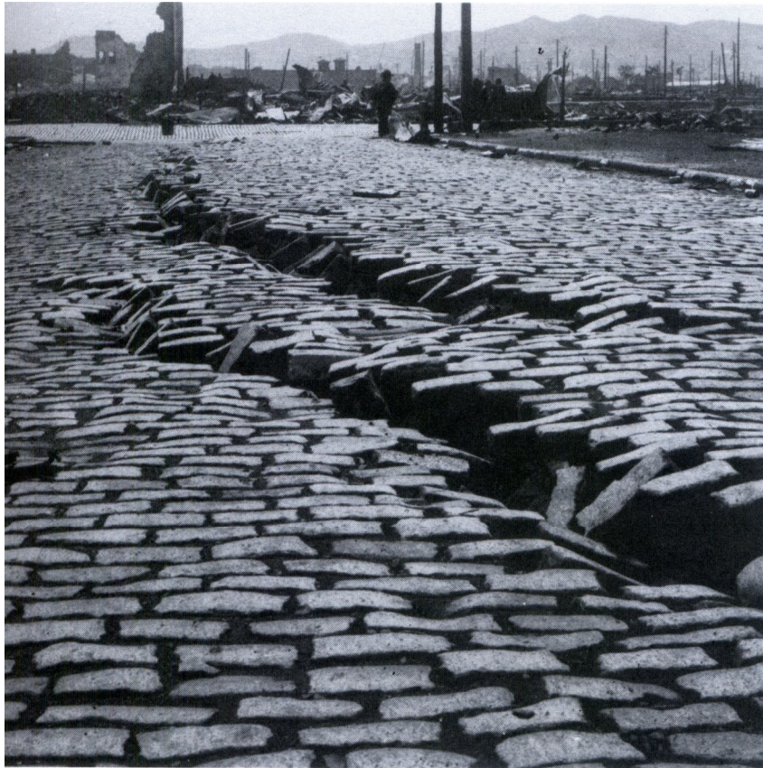
Figure 4.12 Faulting (and fissuring) of a street as a result of the Great San Francisco Earthquake of 1906. (Photograph of Bluxom Street, near Sixth Street by G. K. Gilbert. Courtesy of United States Geological Survey.)
